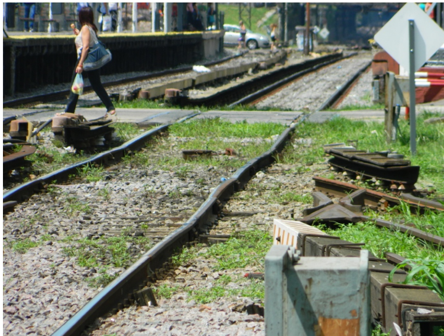
Figure 3: Undulated rails in Caballito station. Photo by author.
